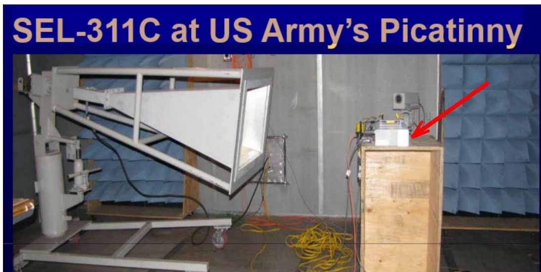
Figure 11: Testing of stand-alone SEL-311C (marked by arrow) DPR by exposing it to a directed high-frequency signal on the test-bench of US army's Picatinny fire range.
