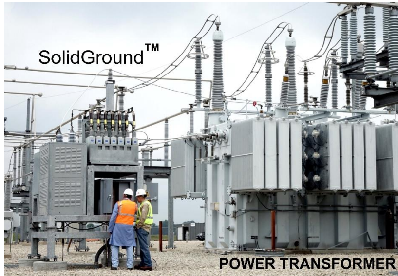
Figure 12: GIC limiter for a transformer's neutral conductor SolidGround™ offered by ABB company
