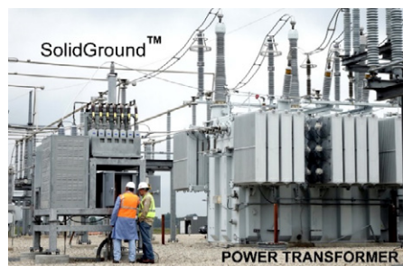
Figure 6 SolidGround™ by ABB (left) meant for blocking GIC in a neutral conductor of power transformer (right)
