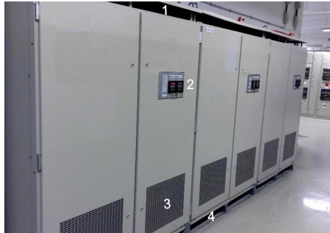
Fig1. Design of power plant's BC. The figures indicate the “weaknesses” of cabinets that allow unobstructed access of HEMP inside the cabinet.
