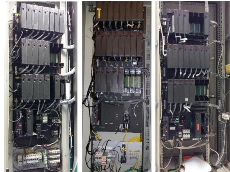
Fig. 1b. MOSCAD-RTU cabinets
