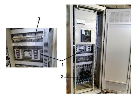
Fig. 26. Complete control cabinet with a microprocessor-based protection relay, filters and DIN-rail surge arresters. 1 - described above filters; 2 – addition filters; 3 – special surge arresters
