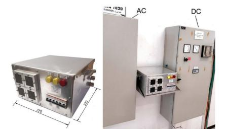
Fig. 29. Automatic HEMP protected charger for auxiliary DC power supply systems of critical infrastructures
