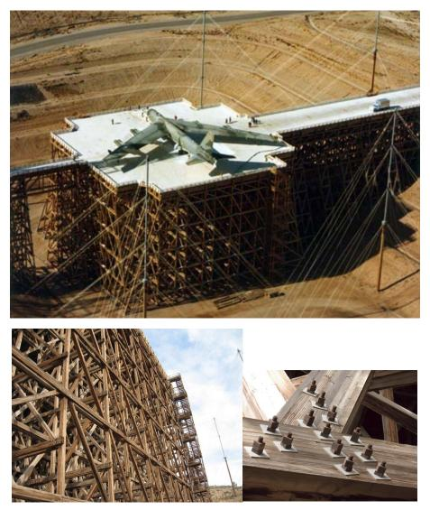
Fig. 18. The ATLAS-1 (Trestle) EMP test facility at Kirtland Air Force Base with a B-52 in test position
