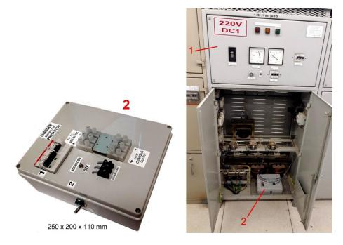
Fig. 30. Charger disconnection module
