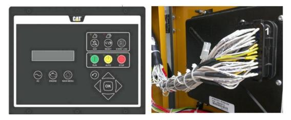
Fig. 35. Main controller of diesel generator
